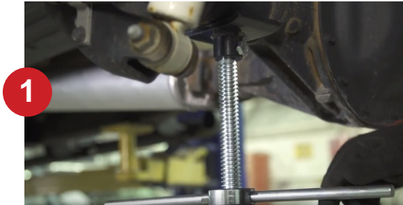
1 Support the rear axle with a jack and jack stands.
